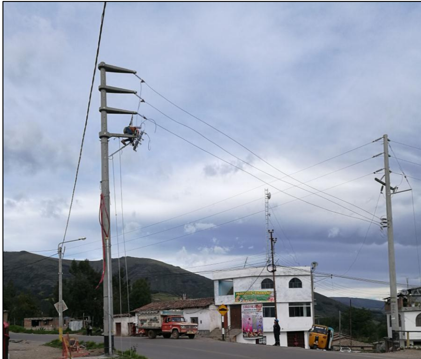
Figura 7: Conductor ACCC 70 mm 2 .
