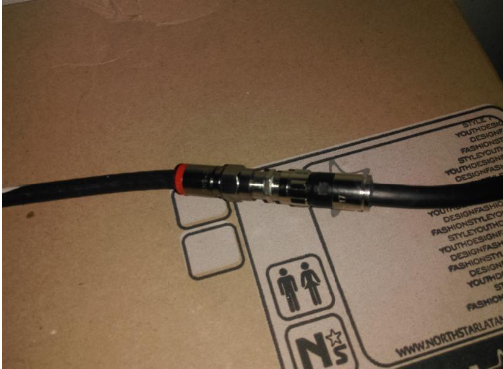
Figura 7: Empalme de cable coaxial
