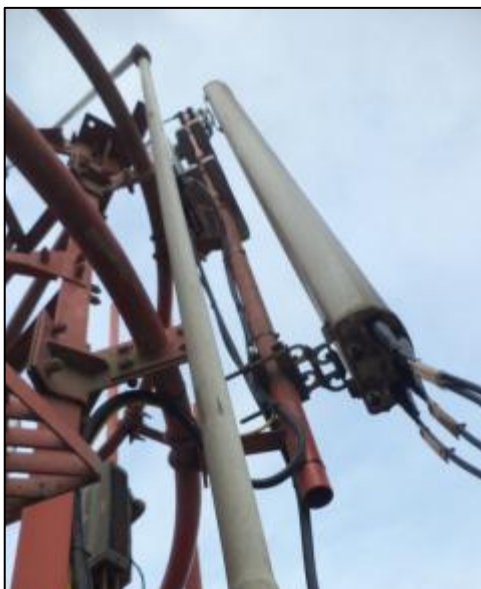
Figura 5.20: Antena COMBA ODV-065R18J18J
