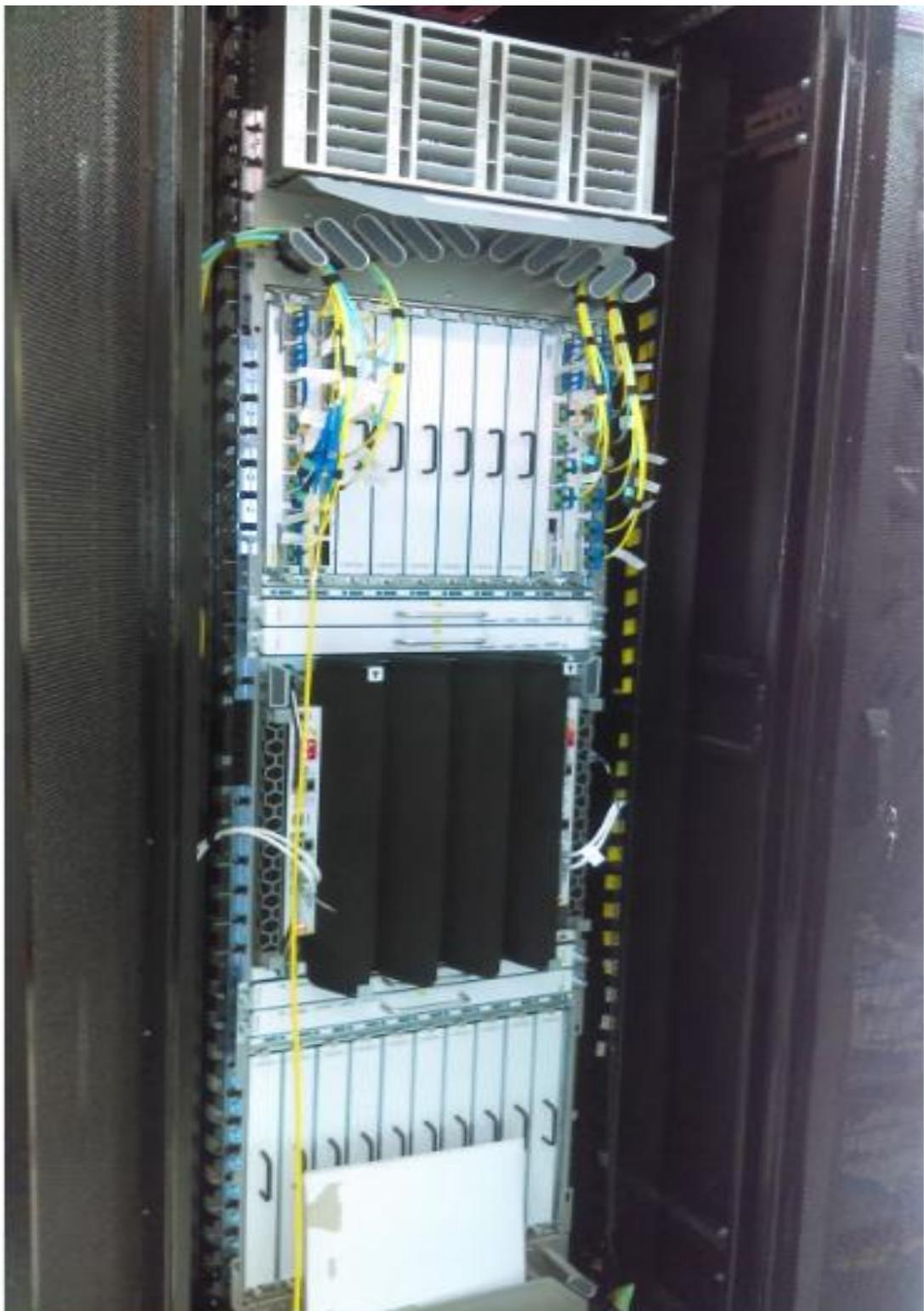
Figura 27: Router Cisco ASR9922
