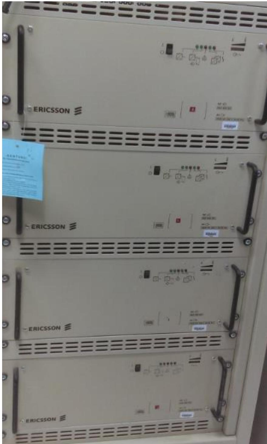
Figura 24: Inversores Emerson Entrada=-48VDC y 2500VAC.
