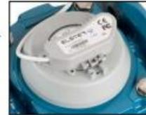
Remember to remove the foil tab before fitting the pulse unit to the meter!
