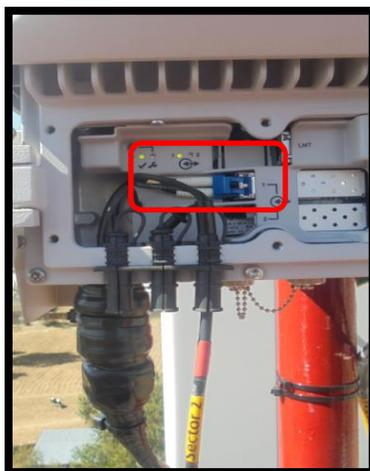
**FIGURA 3-29:** CONECTORIZADO DE LA FIBRA ÓPTICA EN LA RRU.
