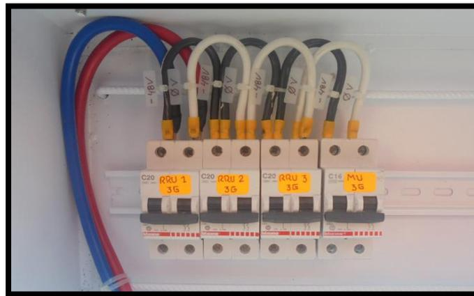
**FIGURA 3-7: CAJA BY PASS PARA ENERGIZAR LA RED UMTS.**
