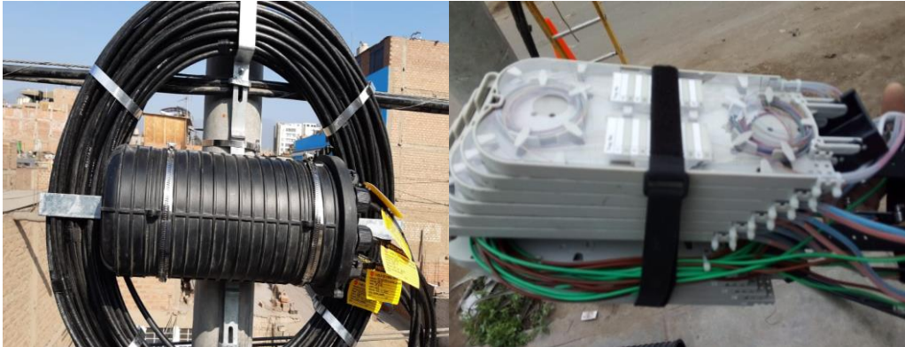
Figura 19. Vertical splice closure
