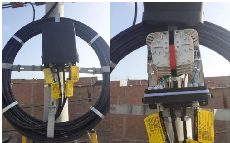
Figura 18. Horizontal Splice Closure 48
