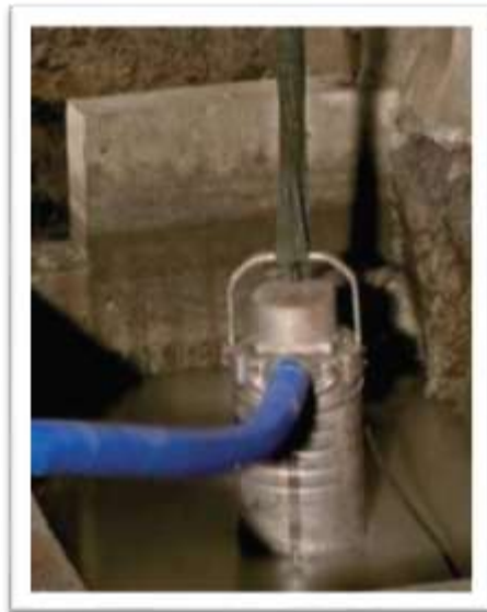
Figura N°34: Bomba sumergible.
