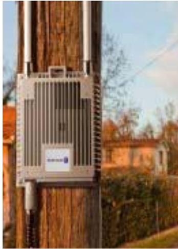
**Figura 13.** Metro-Cell Exterior 9364 1900- 850MHz Alcatel-Lucent.
