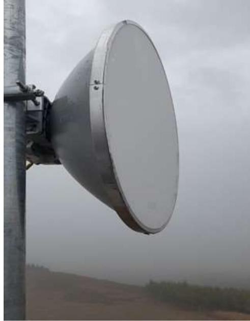
Figura 2.23. Antena Ceragon FibeAir IP-20S.
